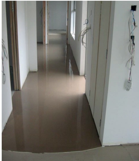
Self-Levelling compound covering elements
