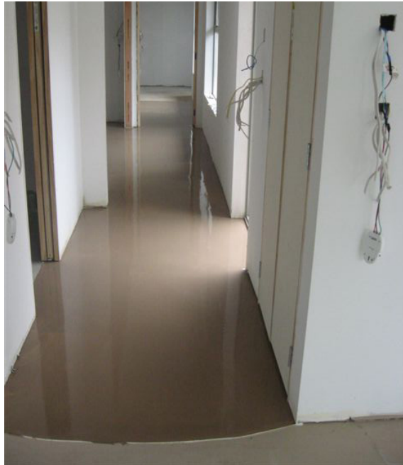
Self-Levelling compound covering elements
